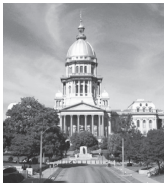
State Capitol Building
